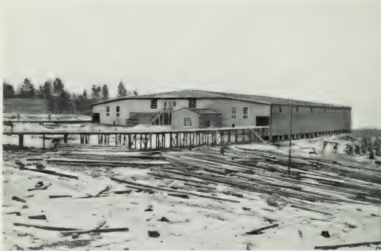
FIG. 130. PROGRESSIVE ARTIFICIAL SEASONING PLANT. [By courtesy of Sturtevant Engineering Co., Ltd.]
